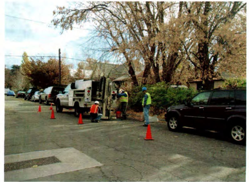
East Side Springs View: East 11/14/11 URS setting up the direct-push unit at 910 E. Harvard Avenue. DERR abandoned the location after meeting refusal at 27 feet bgs. (Photo: MWH)
