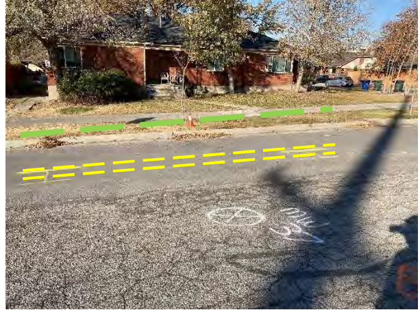
MW-37, gas and sewer (located in the grass parallel to the roadway) located and marked.
