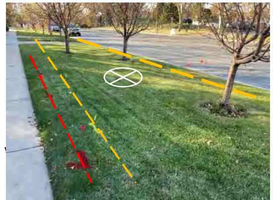
GW-52, Communication running along the road, gas and power between the sidewalk and GW-52.
