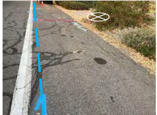
Water line located running up the street adjacent to planter where GW-20 was located in the planter area.
