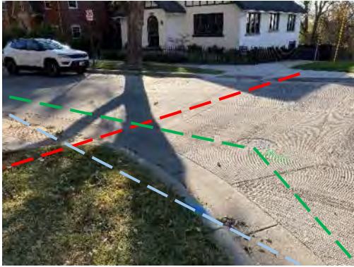
Water, sewer and power near intersection near proposed work area for GW-53.
