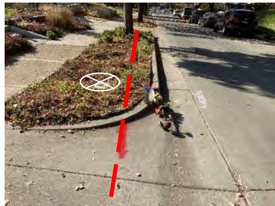
Electrical lines in planter near proposed work area for GW-61
