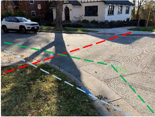
Water, sewer and power near intersection near proposed work area for GW-53.
