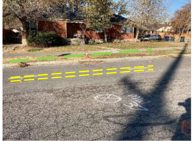
MW-37, gas and sewer (located in the grass parallel to the roadway) located and marked.
