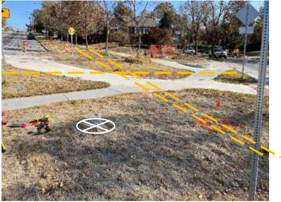
GW-10, multiple communication and sewer lines nearby proposed location.
