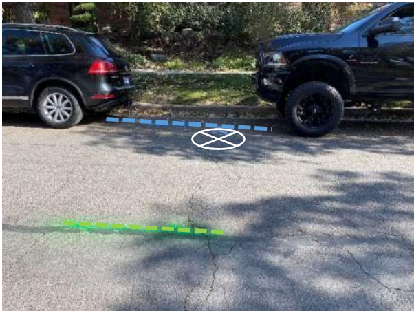
MW 38 (Elizabeth Street option) note proximity of water line markings. Sewer in center of street, recommend engaging Blue Stake before proceeding.
