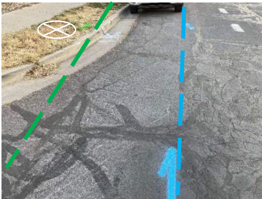
Water and drain lines near proposed work area for GW-59.
