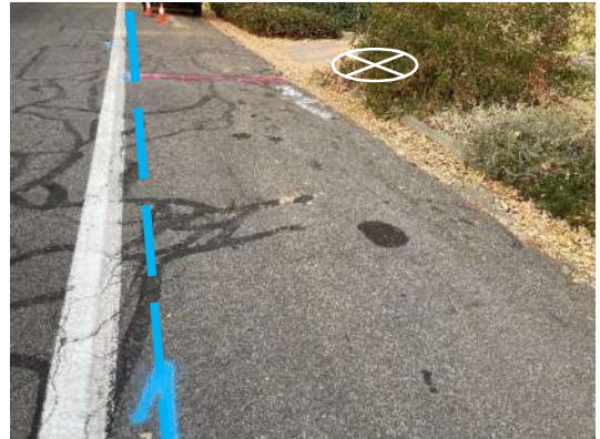
Water line located running up the street adjacent to planter where GW-20 was located in the planter area.
