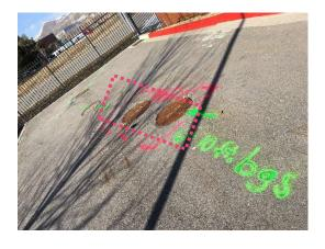
Oil water separator and drain lines near proposed work area for MW-30.
