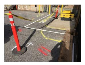
Natural Gas and Propane lines as well as power and communications near proposed location for MW-24.
