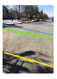
Gas, ~60" sewer line and water lines to the East of proposed work area for MW-32.
